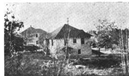
DOUBLE WALL COTTAGES AT LUDLOW, MASS.
